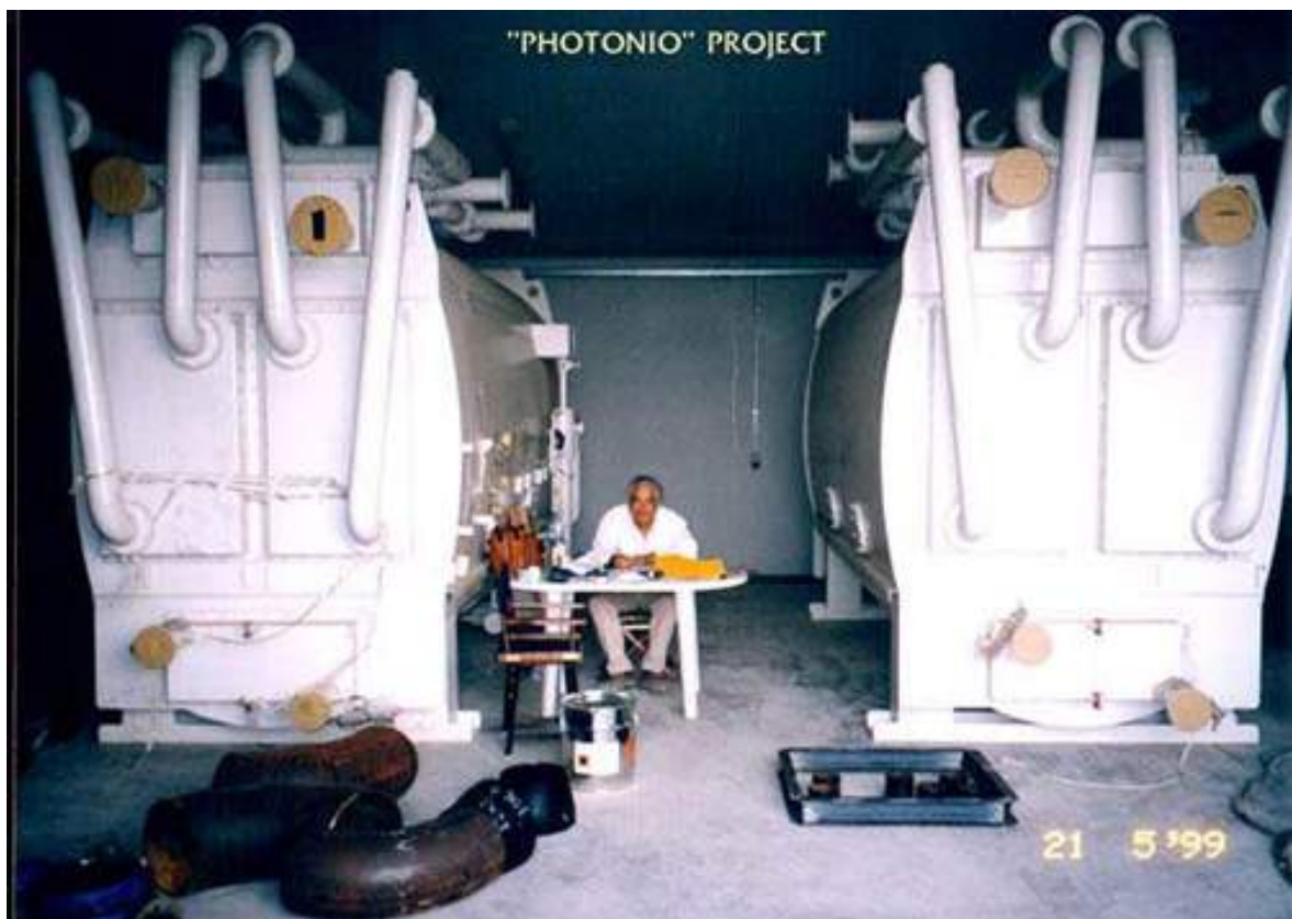
Figure 2: Solar adsorption chiller, Sarantis S.A.
